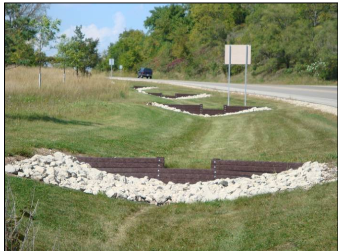
Existing stormwater “runoff ladders”
