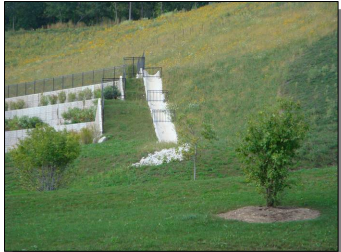
Existing stormwater “runoff ladders”
